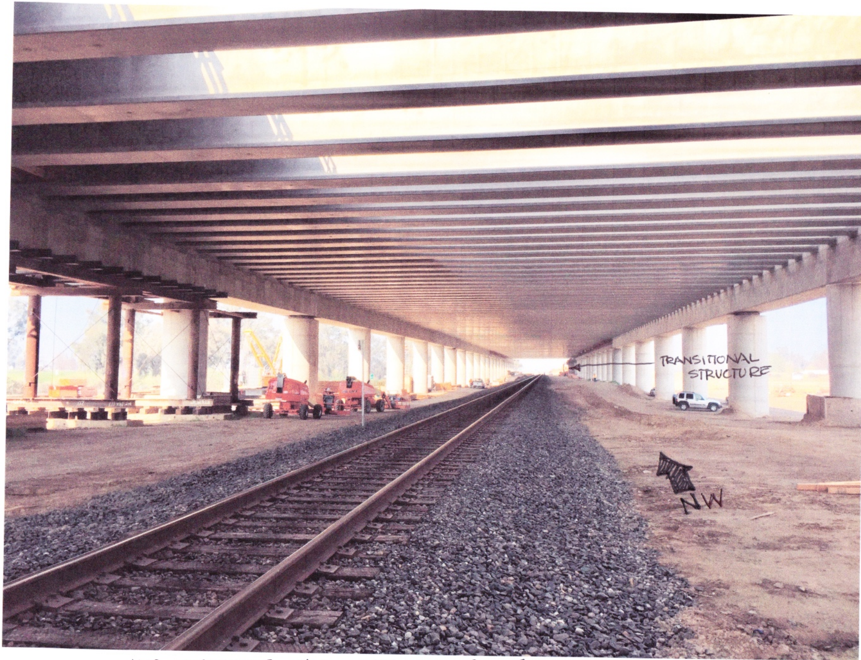
HSR STRUCTURE OVER UPRR TRACKS NEAR HERNDON DRIVE, FRESNO LOOKING NORTHWEST
